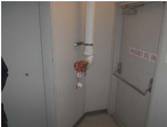
Stairwell and Outside Emergency Door
