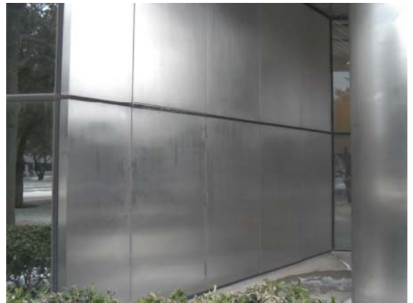
Outside Exit door
